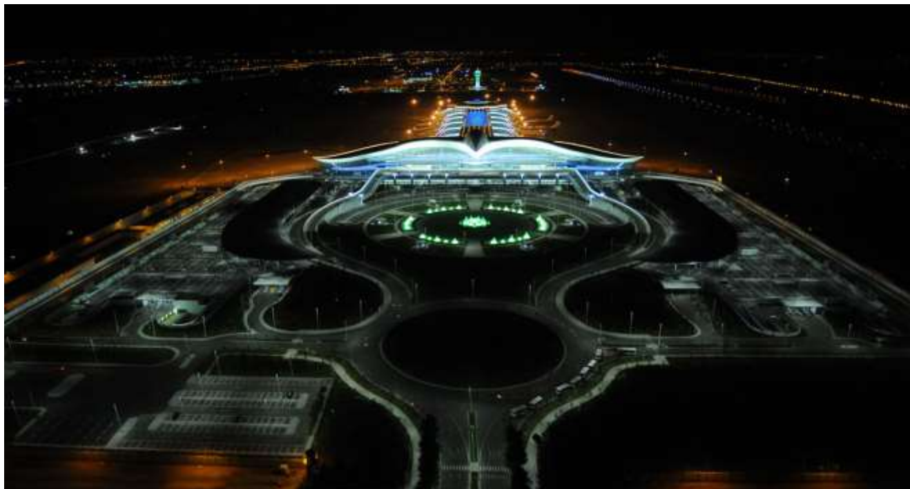
Ashgabat International Airport.
